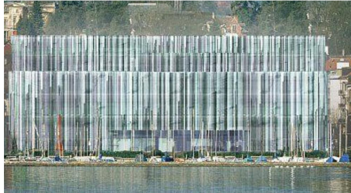
SwissRe (Building NEXT & 5 others)
