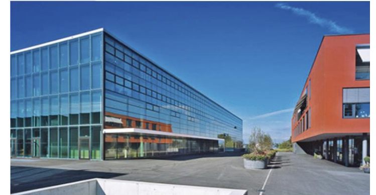
Zug Cantonal Hospital (isolation room)
